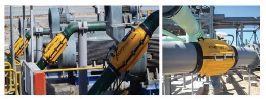
**Smart Technology.** Buckman acquired CCMI and with it came an entrained air technology that has been rebranded as ECHOWISE, which is non-intrusive, provides real-time continuous data and requires no downtime to install. The reliable data it provides enables pulp and paper manufacturers to reduce the amount of variability in their manufacturing process.
