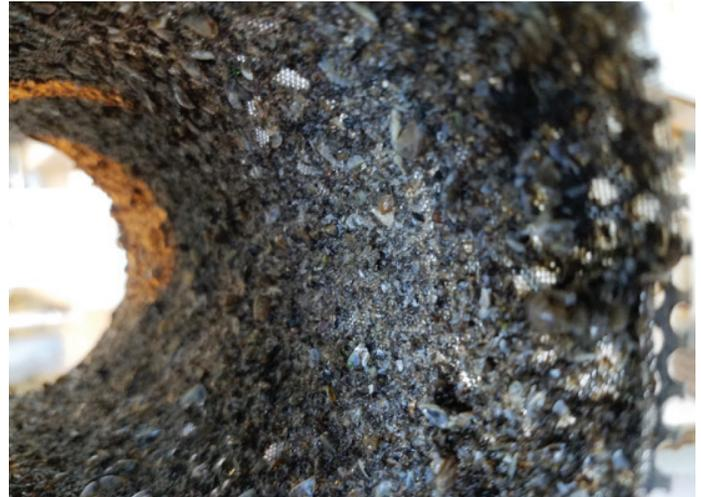
*Figure 2: The vacuum pump heat exchangers filters were plugged with Zebra mussels.*
