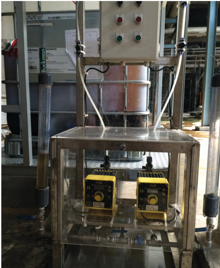
Figure 7. A Maximize® feed system for a two-ply paper machine
